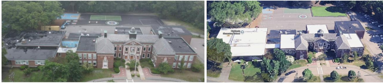
The photos above depict the roof replacement at Braintree's Highlands Elementary School serving 5,809 students. The project replaced partial sections of roof with a new PVC membrane roof, thus extending the useful life of the 95-year-old building. The project reached Substantial Completion in September 2023 and received Final Audit Approval at the December 2025 Board of Directors meeting.
